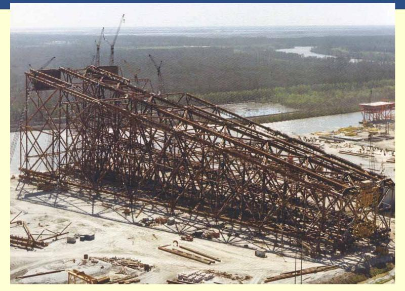
Height (to top of rigs): 327m; Weight (at launch): 26,000 tonne Base dimensions: 107m x 79m; top dimensions: 45m x 25m
