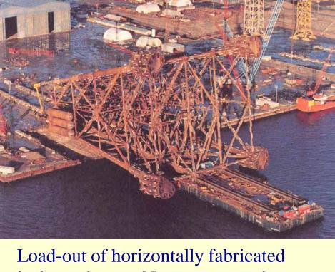
Load-out of horizontally fabricated jacket to barge. Note cranes at the background
