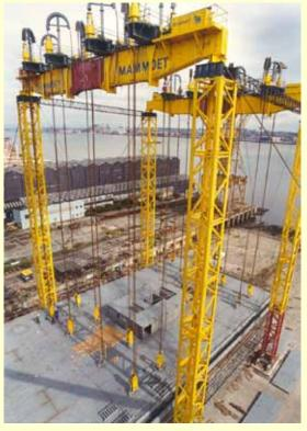
Lifting using synchronised strand jacks
