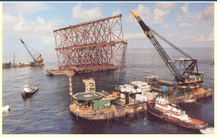
Two crane barges and tugs around mid-section (on transport barge)
