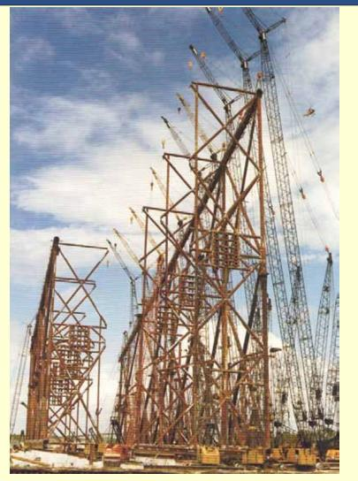
**Reach and capacity of crawler cranes sufficient for roll-up of bent**
