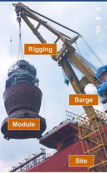
2 stages of lifting lower turret – off quayside & clearing side of Northern Endeavour (Laminaria FPSO)
