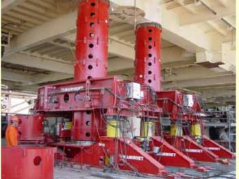
Related to static indeterminacy – Limiting load variation through shimming plates
