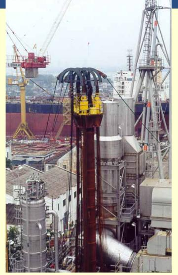
Views of vertical columns and strand jacks prior to lifting
