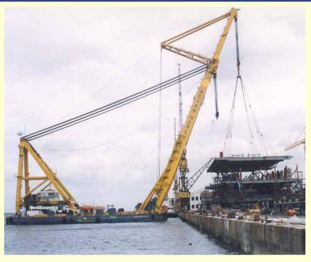
Lifting of deck using strand jacks on columns for placement of loadout truss
