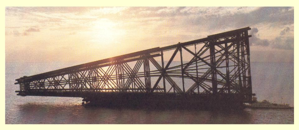
Note the need to check for tow fatigue resulting from large stress ranges imposed on the connections for long and stormy voyage
