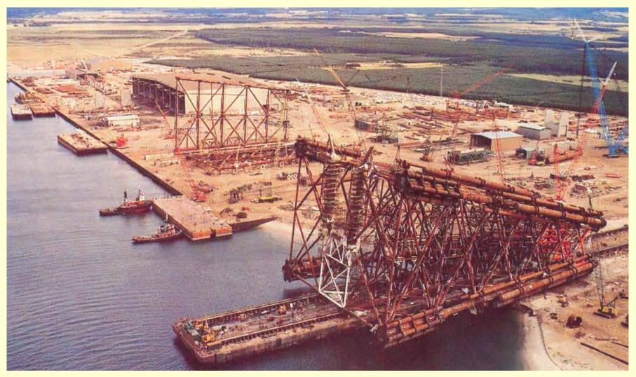
Jacket load-out (in the fore-ground), cranes and flat-top barges
