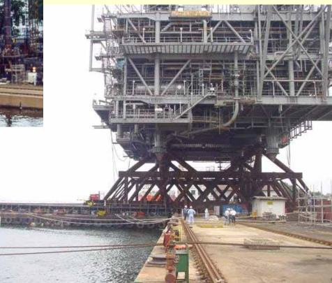
Shell Malampaya Deck – Towing and Placement onto Pre-installed Sub-structure
