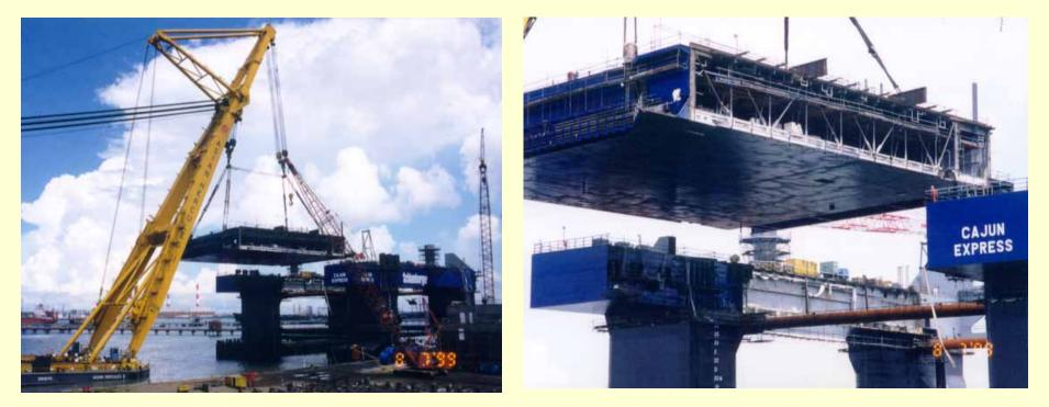
Asian Hercules II sheerleg crane vessel, with centre block, approaching Cajun Express Zoomed-in view (note the temporary truss on side of block, and lift point)
