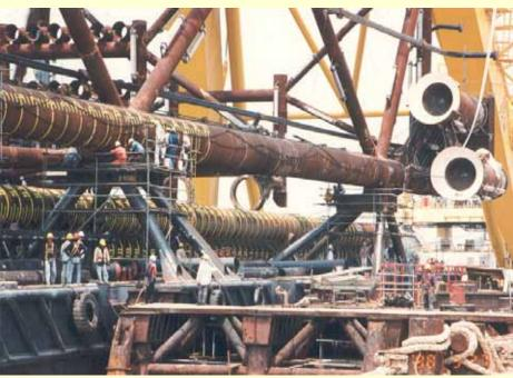
Placement of jacket onto transport barge
