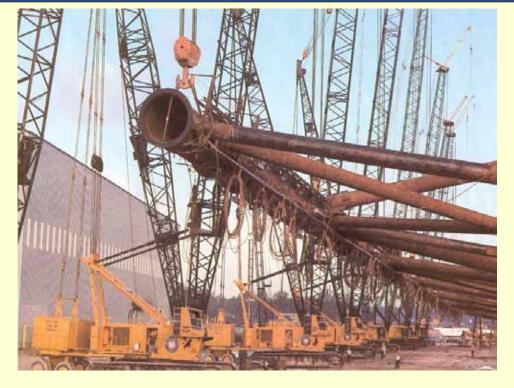
Bent being lifted from horizontal position
