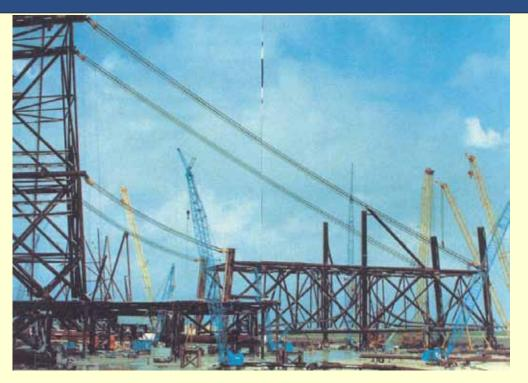
Bullwinkle "core-block" method due to larger dimensions of base structure. At required height, crawler cranes provide <u>in-</u> <u>adequate</u> lift capacity
