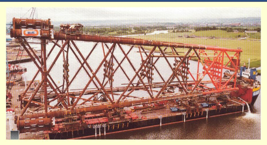
Tie-downs located at jacket and barge strong points (with spreader beam when necessary)
