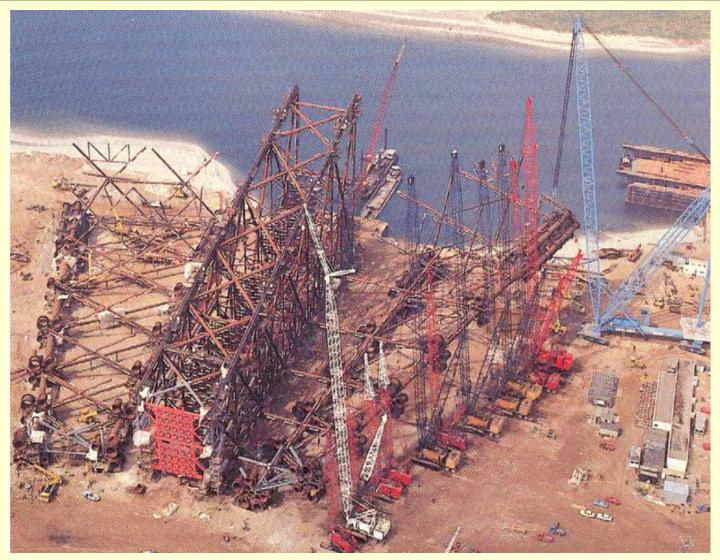
Note the synchronized movement of cranes in the roll-up operation
