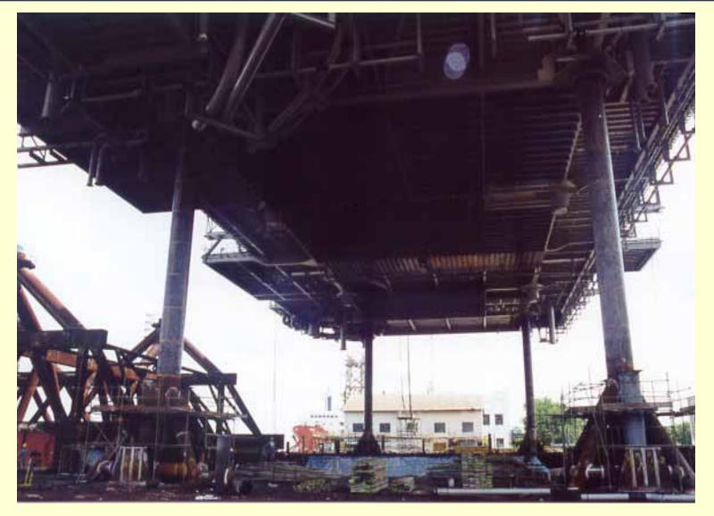
Total deck weight (12,000 tonne) supported on 4 columns
